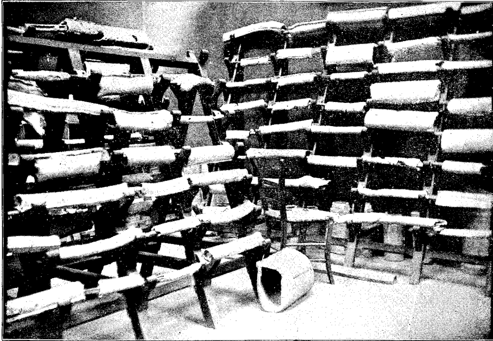
LEAD AND TERRA-COTTA PIPE. 1
